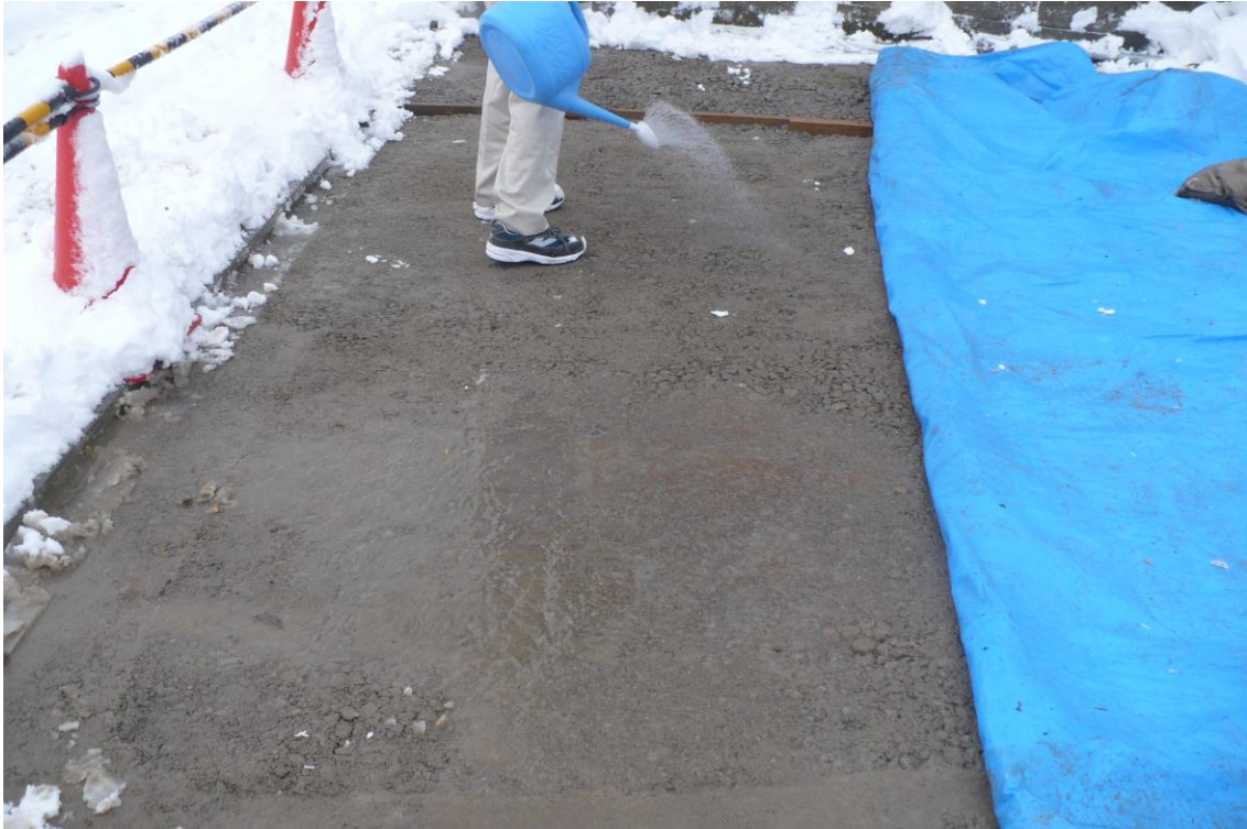
RC40 ATTAC (路盤工法)
